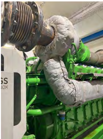
Fig.1: Thermally insulated gas engineFig.
