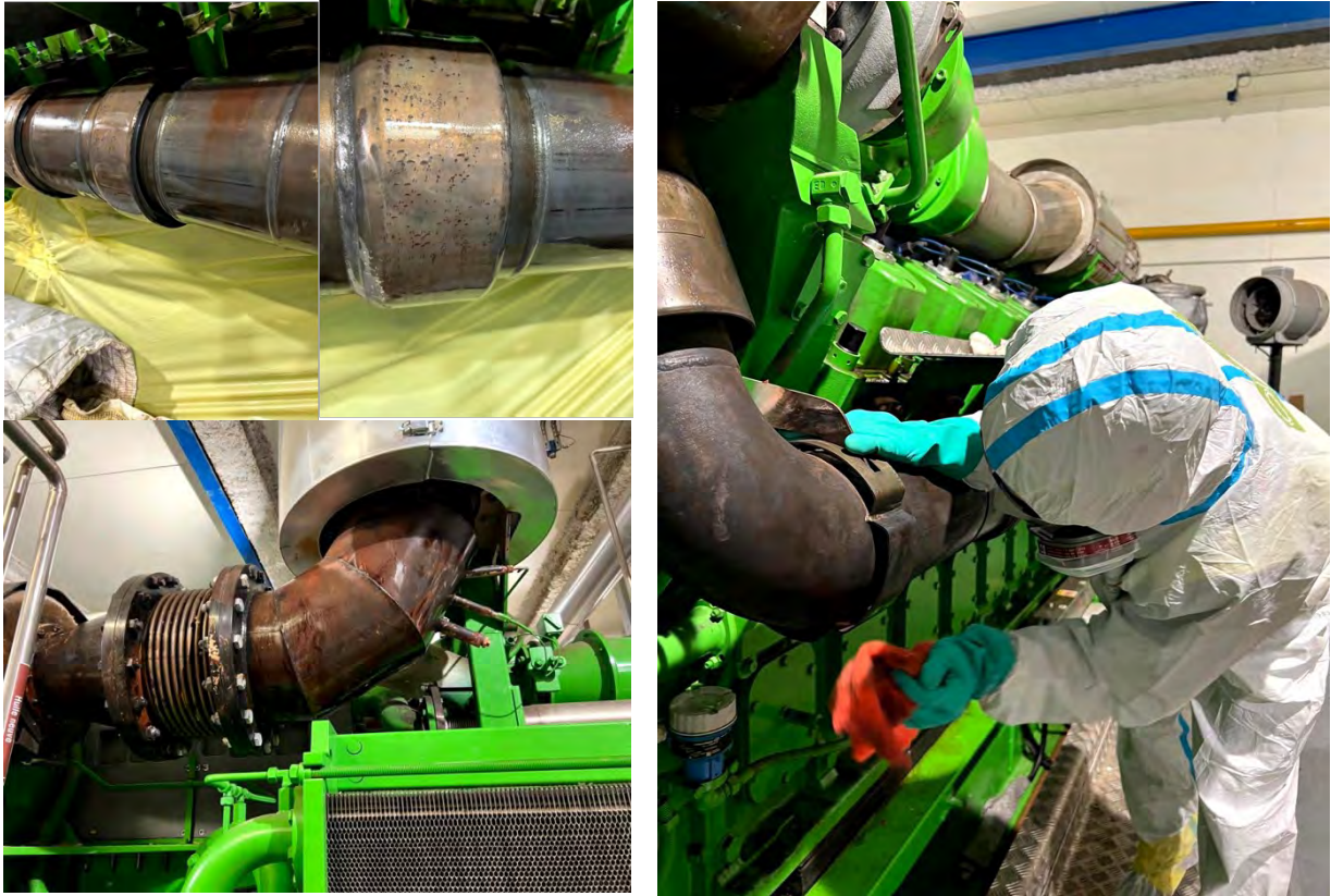
Fig.96-99: Decontamination of system components
