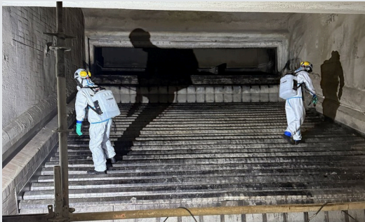
Wetting before starting work on the grate. Full face mask, disposable protective suit with hood, gloves.
